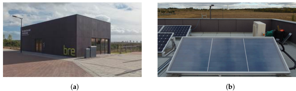
Figure 4. Considered building and corresponding installations. (a) Property. (b) STC and PV installations.
